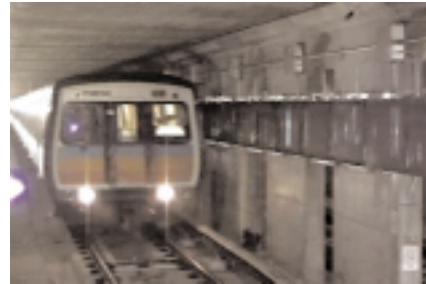
A tunnel in the Metropolitan Rapid Transit Authority system will be the site for innovative advertising.
